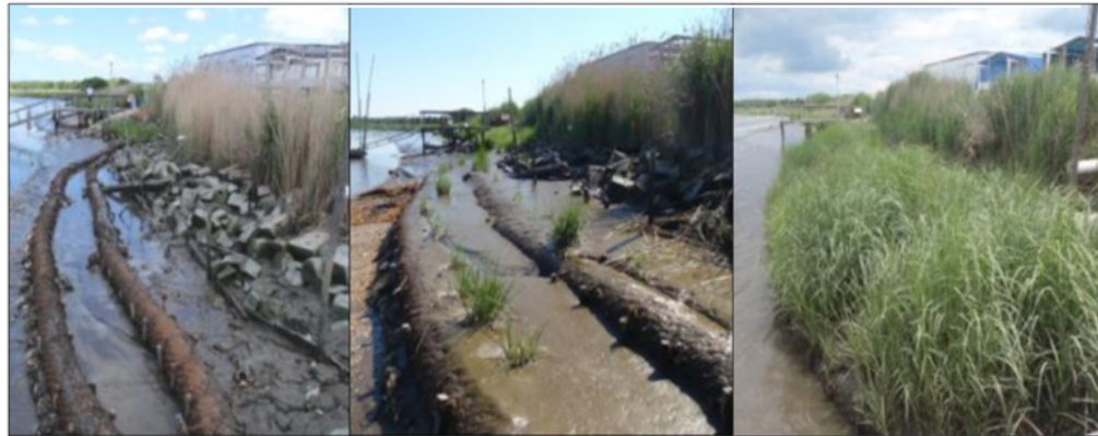
Photo 8: Courtesy of Dr. Josh Moody. Photo showing coir logs stabilizing sediment and supporting vegetation growth at eroded marsh
